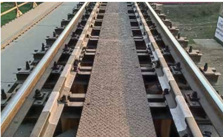
Revitalizing Nalhati Bridge, Eastern Railway – Howrah Division, West Bengal : Evolution from Corrosion-Prone Mild Steel to Enduring Stainless Steel Chequered Plates - Ensuring Longevity and Strength.
