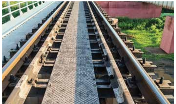
Revitalizing Nalhati Bridge, Eastern Railway – Howrah Division, West Bengal : Evolution from Corrosion-Prone Mild Steel to Enduring Stainless Steel Chequered Plates - Ensuring Longevity and Strength.
