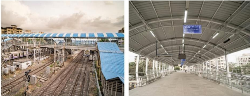
Girders, Columns, Cross Beams etc.
