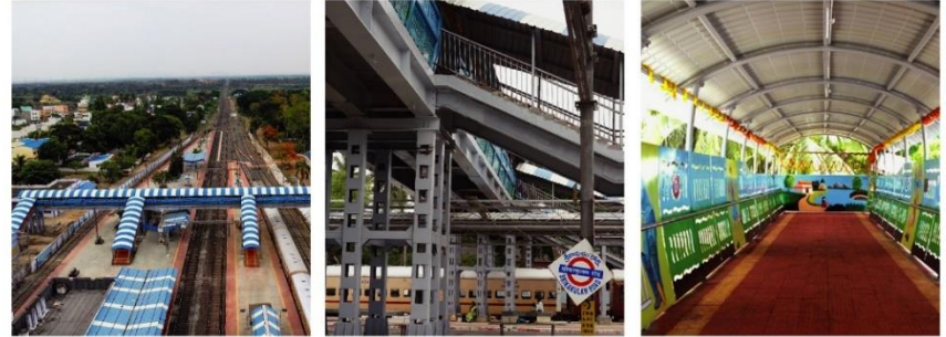
Girders, Columns, Cross Beams etc.
