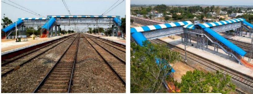
Girders, Columns, Cross Beams etc.
